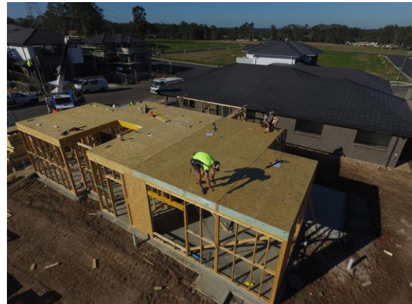
Floor complete – Box Hill
