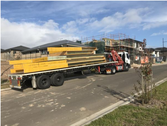
Floor cassettes arrive at site – The Ponds
