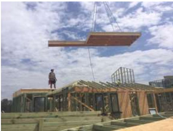
Lifting into position
