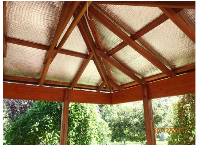
Cantilever Pitching Beams to corner
