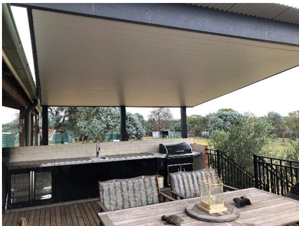
Lining Boards completed
