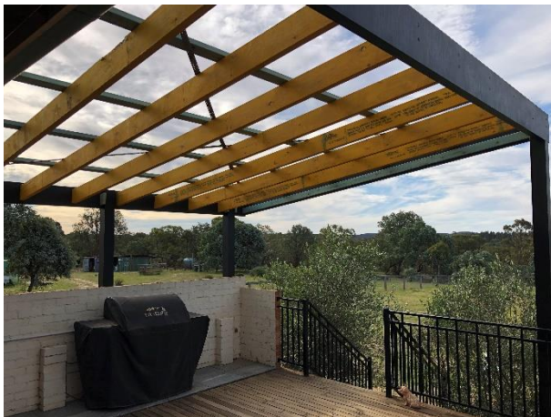
Main Structure Completed
