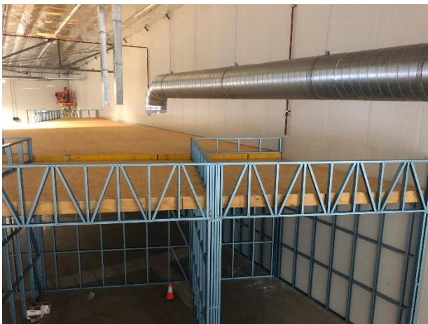
First stage complete
