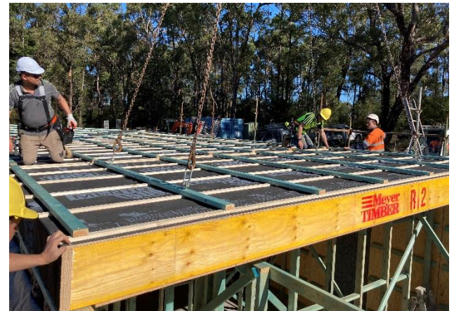
1.5 hour install and ready for sheeting
