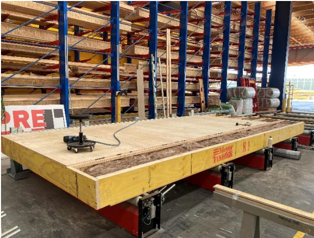
Insulation being installed after underside lined
