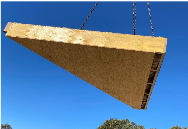
Completed roof cassette being lifted into position
