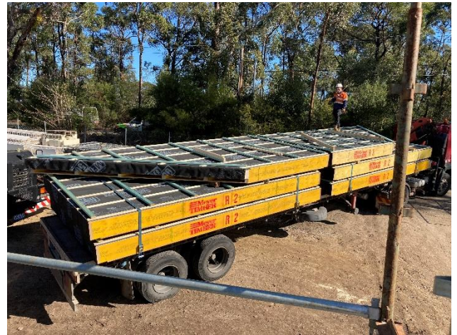
Cassettes delivered to meet crane on site
