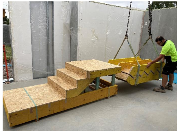
Stair modules staged on site
