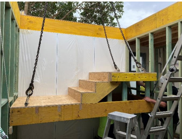
Stair module craned into place
