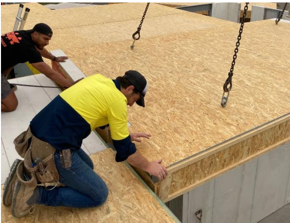
Floor cassette into steel beam
