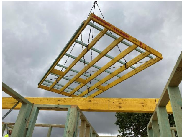
Rafter cassette installation
