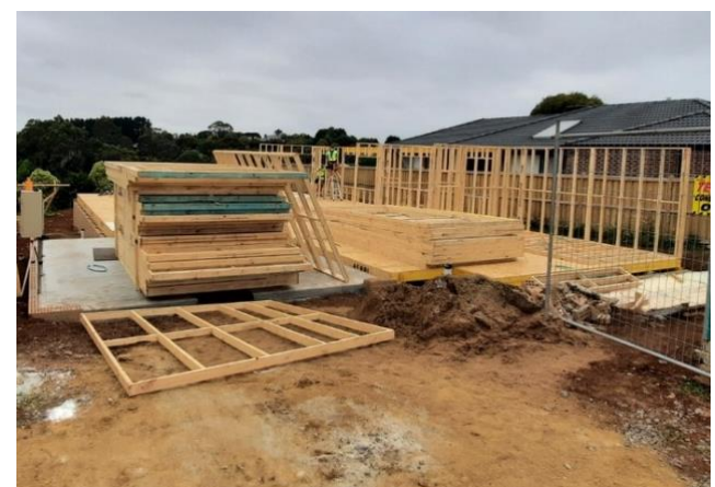
Wall Frames up following morning at 8.30am
