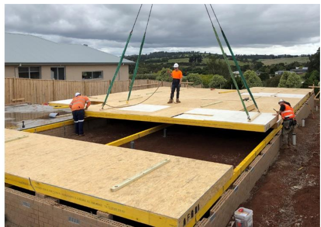
Floor cassettes being installed
