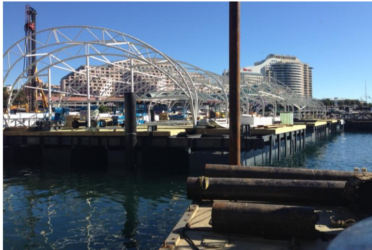
Pontoon finished and in position during fit-out
