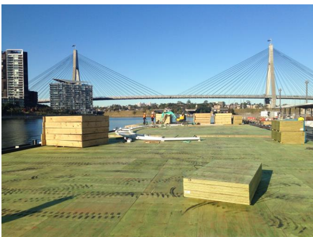
Plywood flooring being installed
