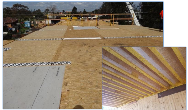
Completed Qikpanel floor system at Level 2
