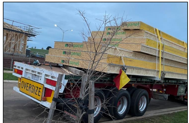
Floor cassettes arrive on site.
