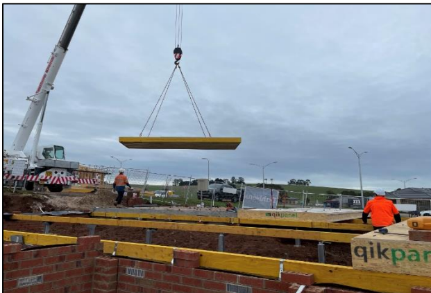
Installation in progress.
