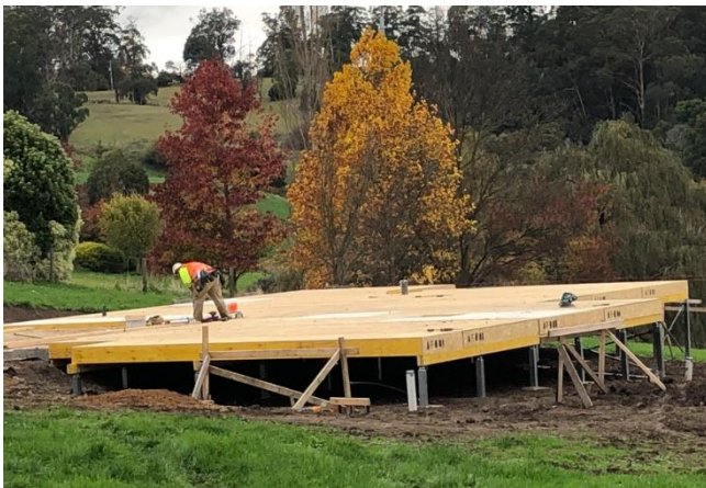
Finishing touches being given post installation.
