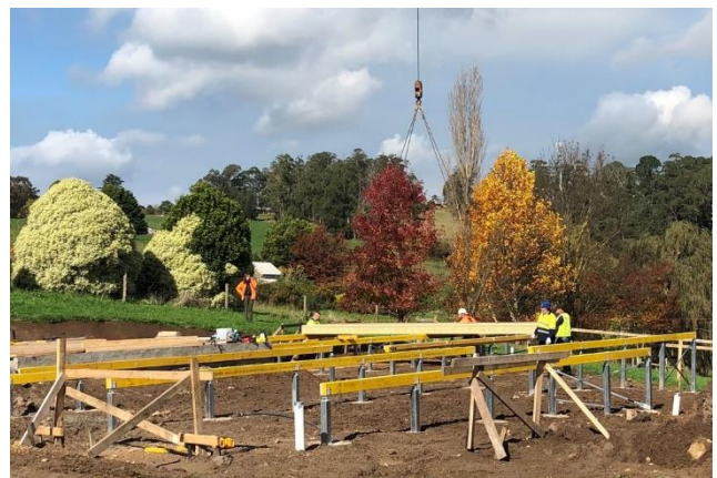
The first cassette installation in progress.
