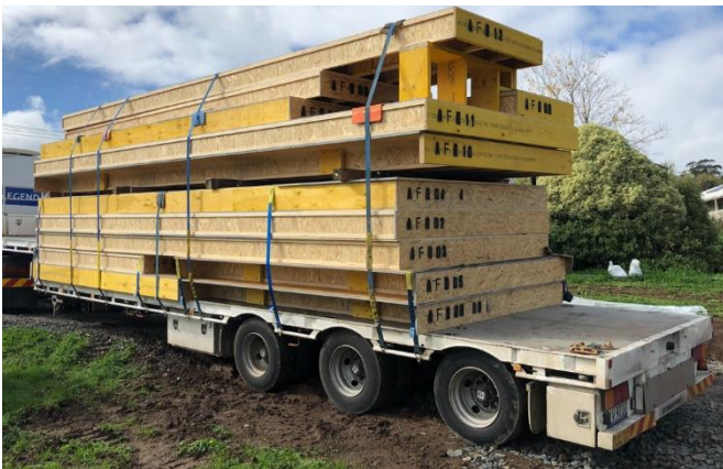
Floor cassettes stacked meticulously to avoid double handling on site.
