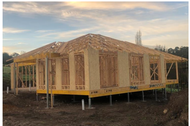
An impressive view of the completed frame and roof truss installation.
