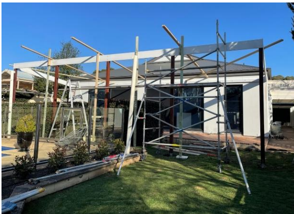
Posts and Beams erected
