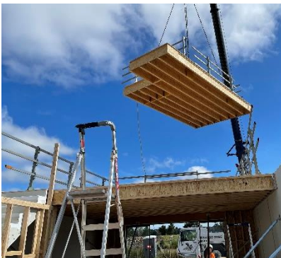
Floor cassettes being installed and roof cassettes in place(right)
