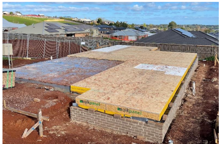
Installation done and dusted
