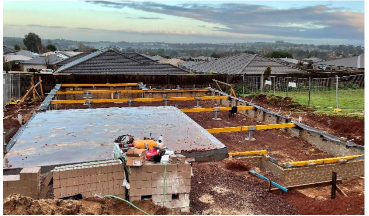
Floor bearers being installed
