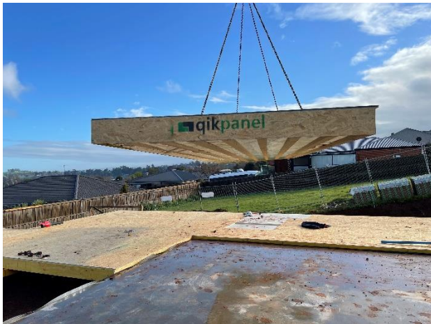
Cassette installation nearing completion
