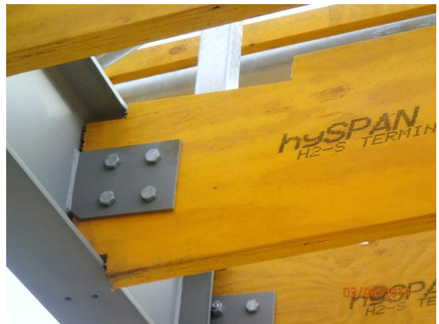
Prefabricated steel beam and box gutter cutout
