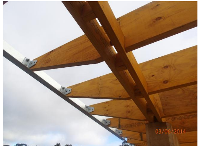
Rafter taper and spaced pitching beam
