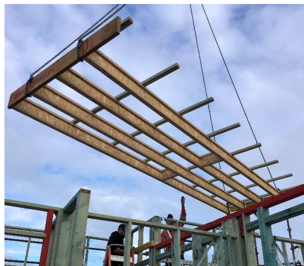
Lifting into position
