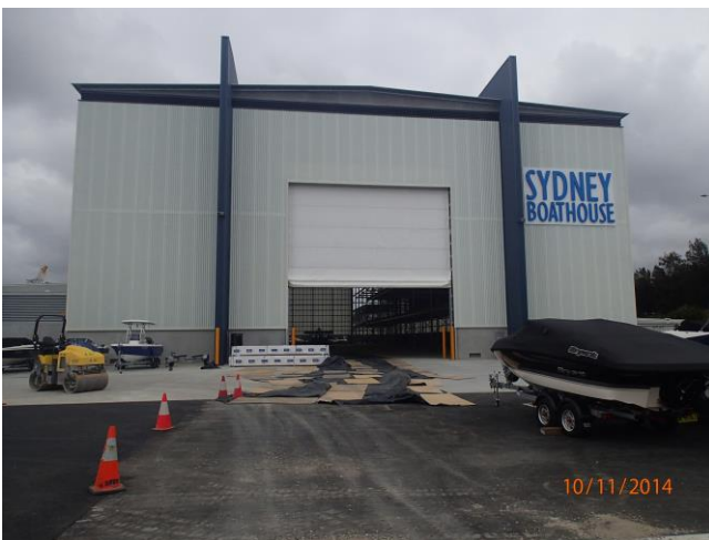
Exterior view of building
