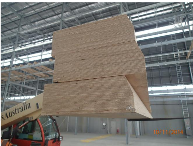
LVL members ready for installation
