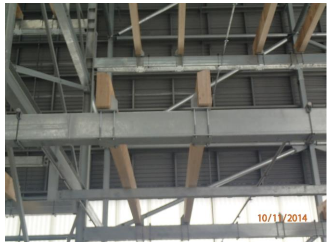
View of boat storage bay
