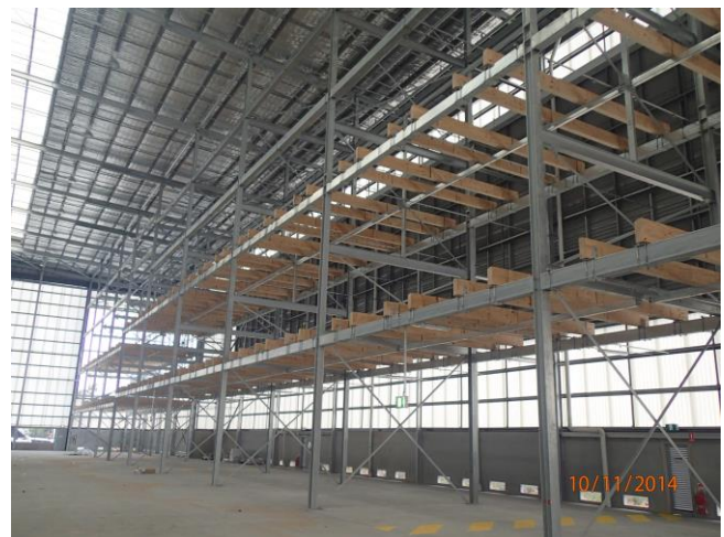
Boat runners installed
