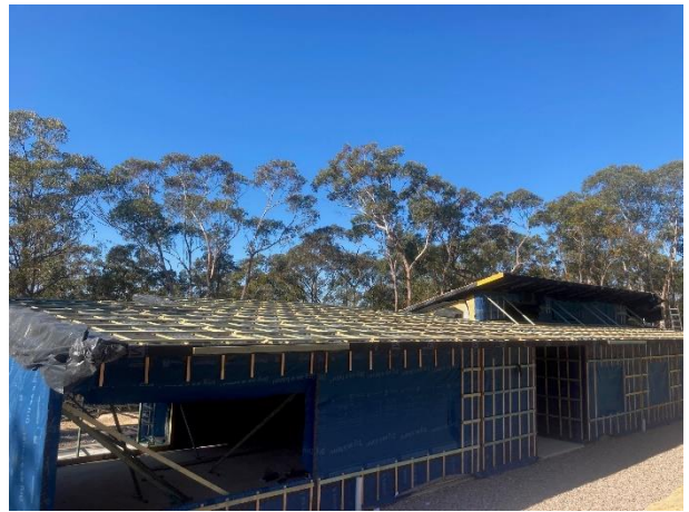
Roof cassettes and wall panels installed
