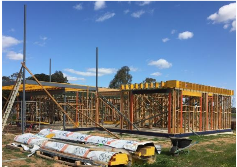
LSL stored on site ready for first floor frames
