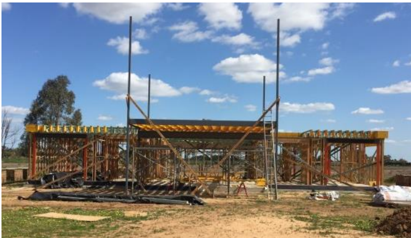
Overall View – Ground Floor
