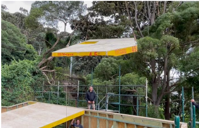
Installation in progress
