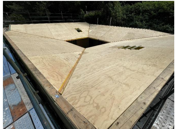
Completed roof ready for battens
