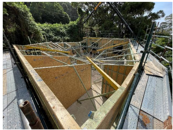
Walls awaiting roof cassettes
