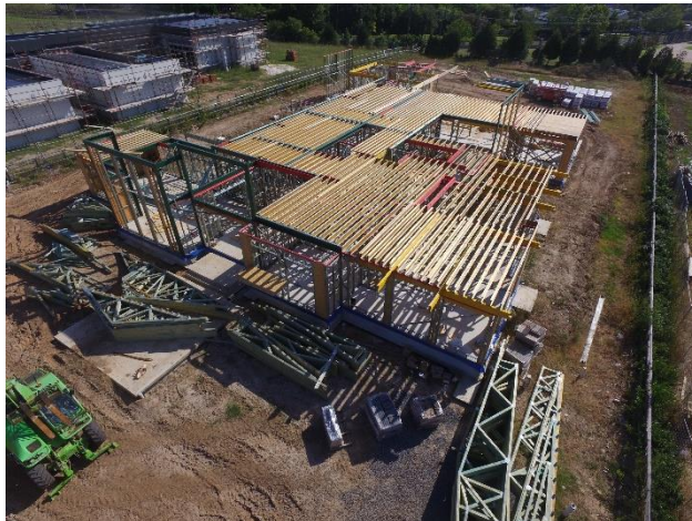
Aerial view showing scale of floor
