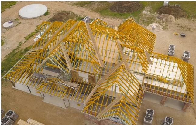
Main Structure Completed
