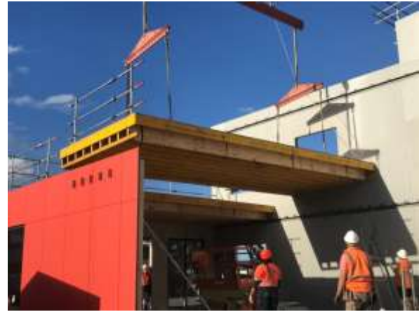
Floor Cassette being installed
