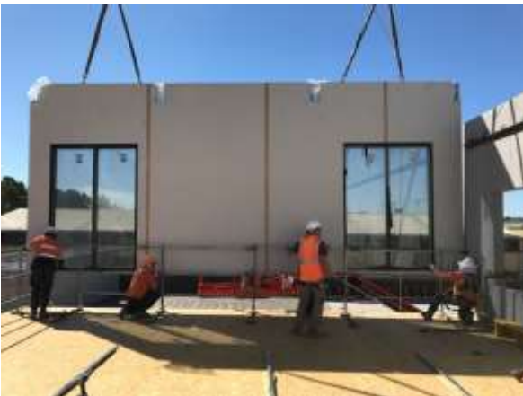
Wall Panel being installed
