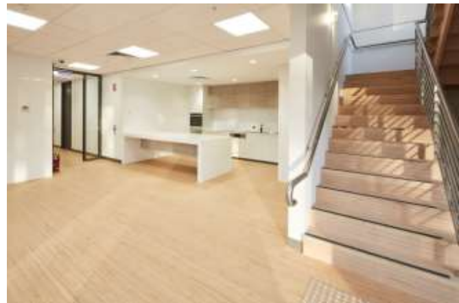
Baubuche flooring and stairs
