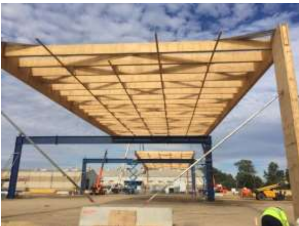
Initial brace bay
