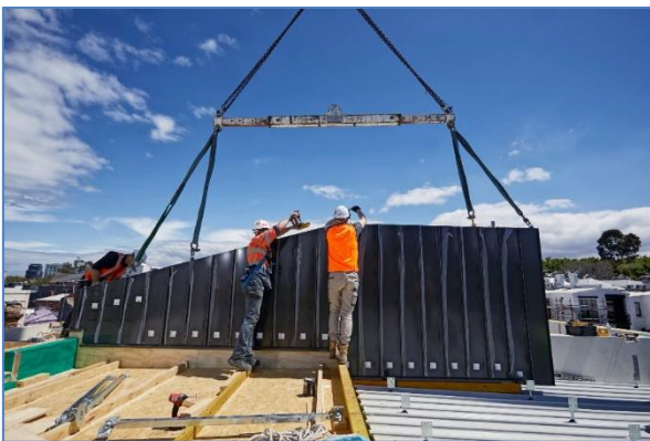
Lifting into position
