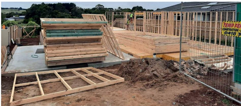
Above: 8.30am (following day) – the floor would usually still be going in, here the wall frames are half up.
