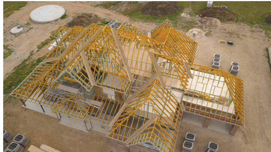
Figure 1 – 3 levels and 49° roof pitch put this building outside of AS1684 requirements
