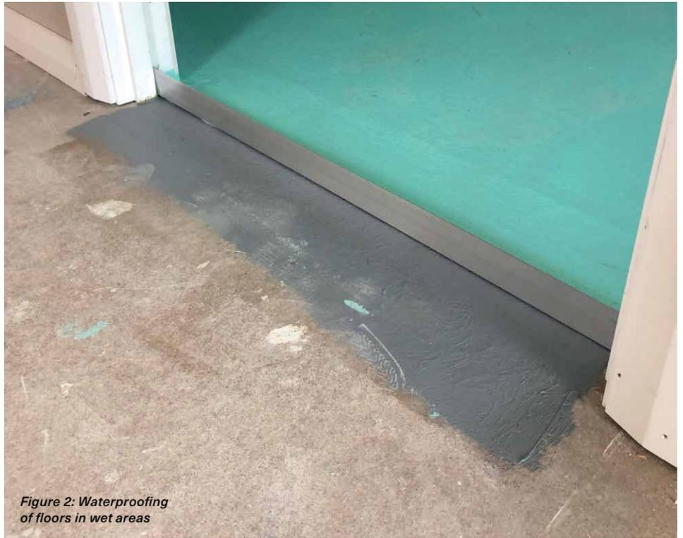
Figure 2: Waterproofing of floors in wet areas
