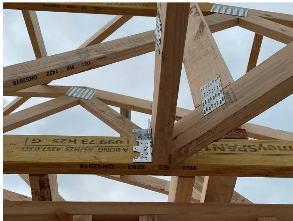
Figure 1: LVL used as the bottom chord of a truncated girder truss.
