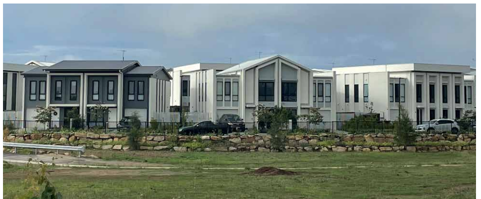
Above: Sunland Developments in Mt Annan, NSW, has 149 units based on only six basic designs. Yet with those limited designs there is still a lot of façade variation.
