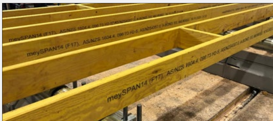
meySPAN14 being used in pre-fabricated floor cassettes at TBS
